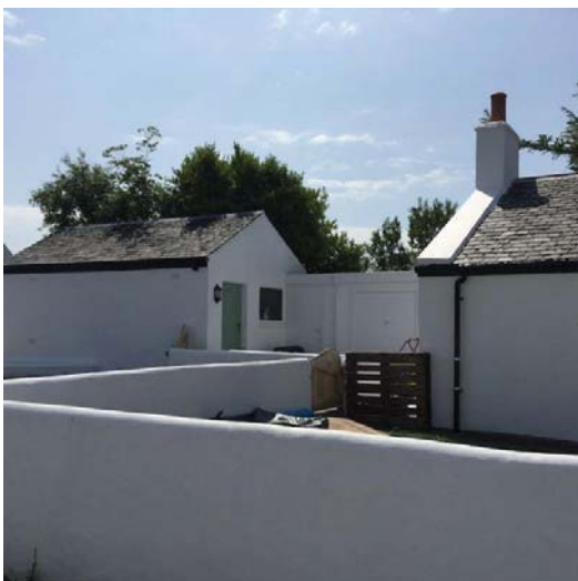
This is the newest major development in the village where Council Officers recently approved the removal of a small existing stone wall, trees and shrubs and replacement with white rendered walls, new white rendered outbuildings and upgrade of white rendered garage.
