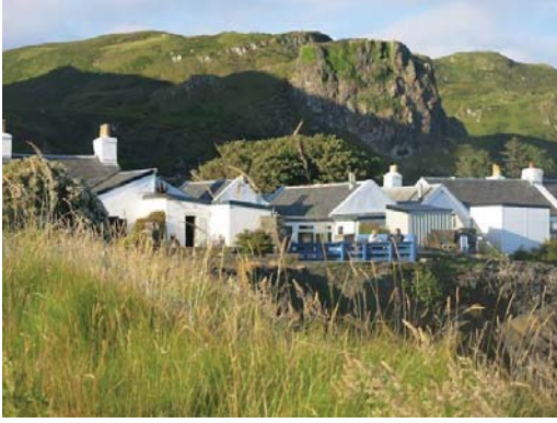
Ellenabeich - South, White rendered shed/store/workshops with black/dark grey roofs. No stone cladding.
